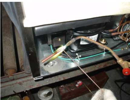
1-4-11、 Install the vacuumizing connector onto the process tube.
