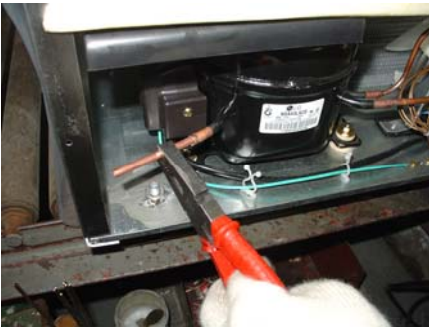
1-4-10、 Weld the process tube
