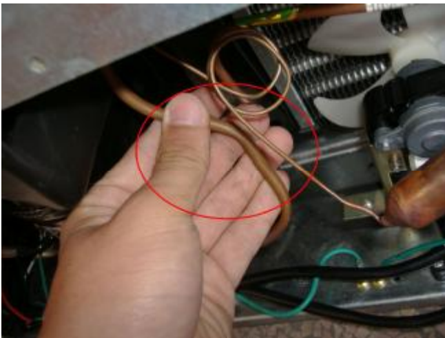
(6)用手触摸回气管，回气管不冷 The intake pipe isn't cool by hand.
