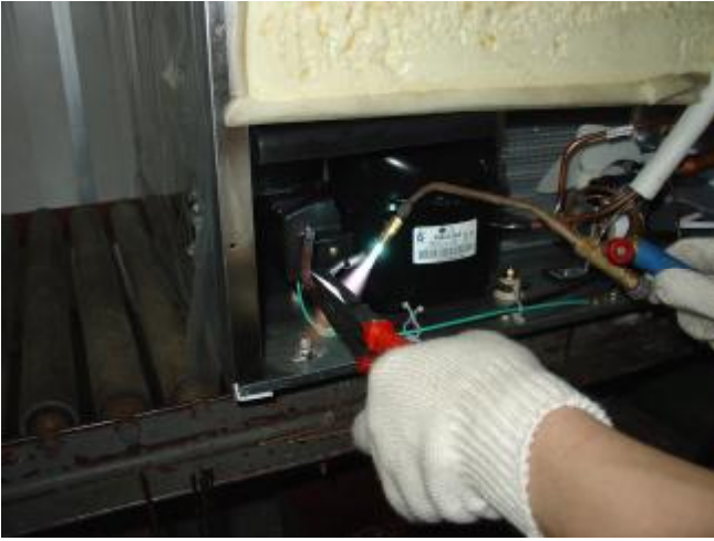
c. 换上新的工艺管 Replace a new process tube
