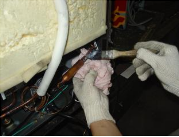
h. 脱开快装接头，用焊枪重新焊接有气泡产生的焊点 Re-weld the parts at which there are seams
